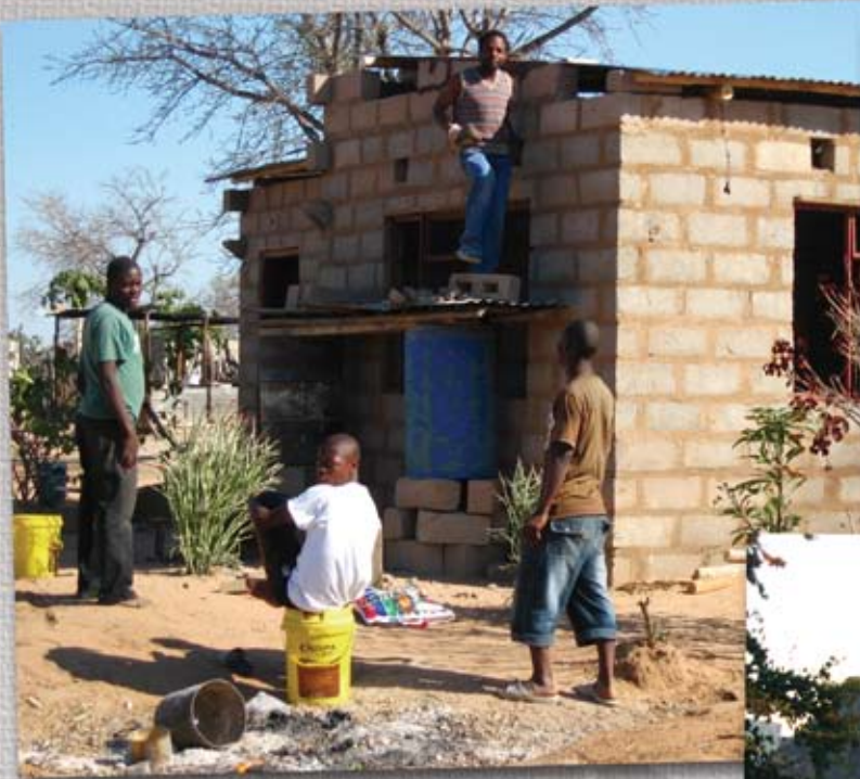
Above: Construction workers adding a new room to a “block standard” house
